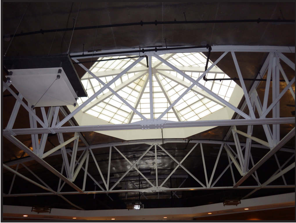
Figure 14. Interior, Steel Bow Trusses
